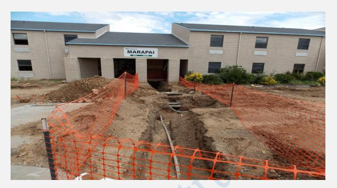
Chilled Water Line fed From Chiller Plant for Marapai Cooling
